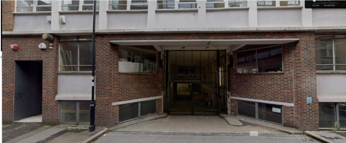
Figure 9: Entrance to basement car park
